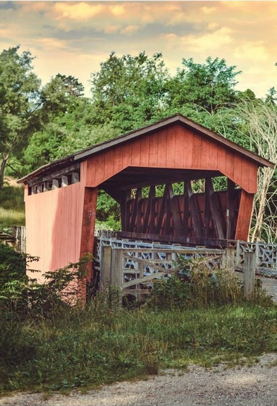
Shaeffer Campbell Covered Bridge-Belmont County
